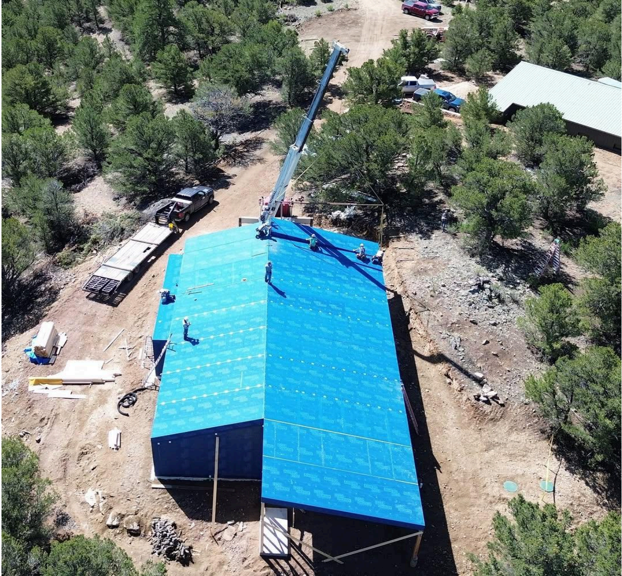
Image credits: Old Country Construction and 475 Supply
